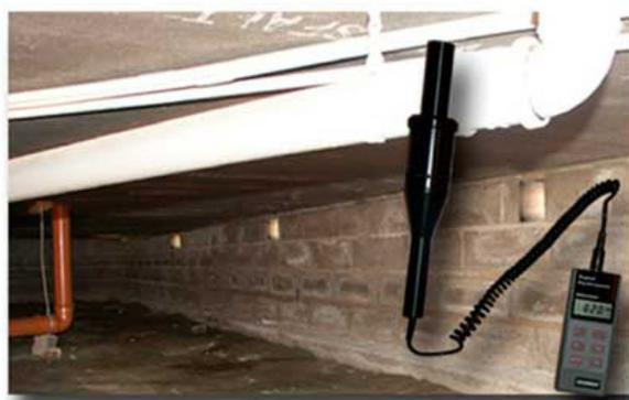
Above picture shows a typical under floor area of a house from the 1980's. Despite of the many vents the relative humidity is fairly high. When the picture was taken, the humidity in the under floor area was 82 % RH and the temperature 12 ° C. Outside the corresponding figures were 62 % RH and 17,5 ° C. With the installation of a **SolarVenti**, the result would have been different. Try, and judge for yourself!
